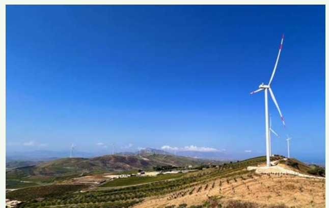
The new system installed in Partinico-Monreale
